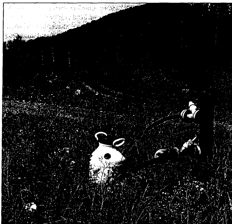
WELLHEADS FOR SUSTAINING HYDRAULIC BARRIER AT STRÁŽ
